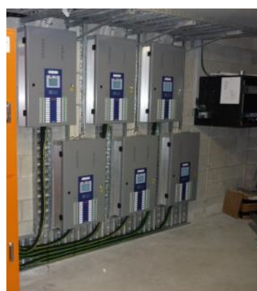
144 channels of EKO installed (Mackay Entertainment Centre)
